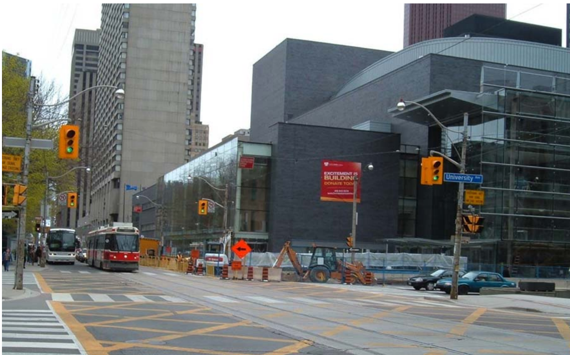
Figure 8 -- Four Seasons Centre for the Performing Arts near the end of construction showing the proximity of rail and heavy vehicle traffic
